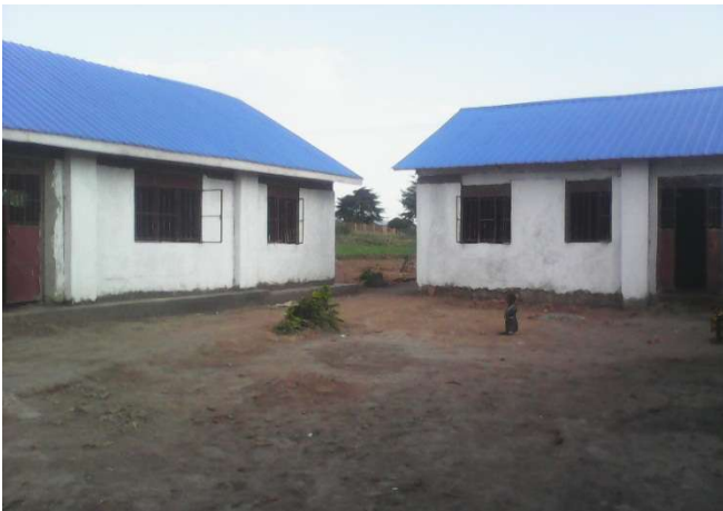
Boys moved in their dormitory (not complete) , funded by German Embassy
